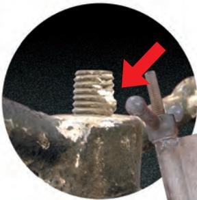
Seized wing nuts and galled bolts that will not operate make simple maintenance and gasket replacement difficult if not impossible.
